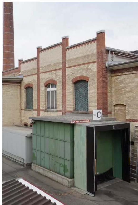
Delivery docks have been added to the monumental building of the Schlachthof—now being used by the Metzgerei Angst.
