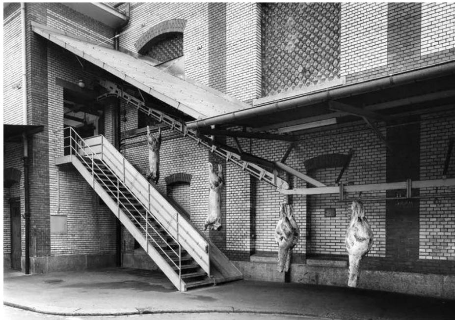
Slaughtered bodies carried over stairs to the exterior by the transport rail, slaughterhouse Zurich, 1960. Photograph: Erwin Kuenzi. Source: Baugeschichtliches Archiv der Stadt Zürich
