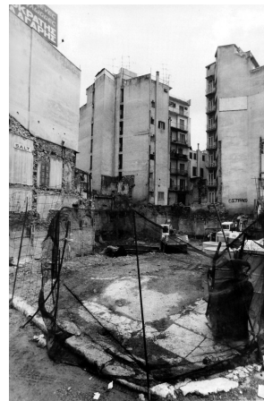
Manolis Baboussis, Construction Site . Source: Athens: 1985 -1996, M. Baboussis personal archive.
