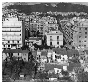
An Inner City Squatter's Settlement in Athens, 1966. Source: Dimitris Philippides, “Town Planning in Greece”, in 20th Century Architecture in Greece (New York: Prestel Publishers, 1999). Courtesy of Dimitris Philippides Archive. 1. Cornelius Castoriadis, “The rationality of Capitalism”, in Figures of the Thinkable , trans. Helen Arnold (Stanford: Stanford University Press 2007), p. 55. 2. Ibid. , 54.
