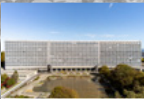
ILO Renovation 2015 - 2019 300 Mio. CHF
