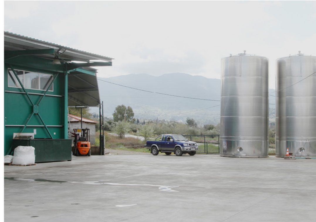
Exterior view with bioenergy silos
