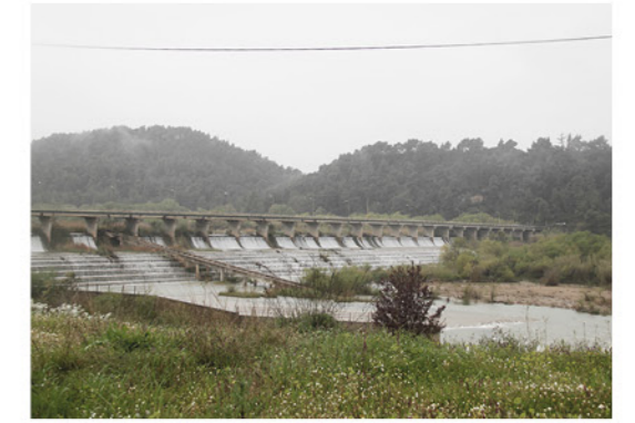
17 The dam of Alfeios River
