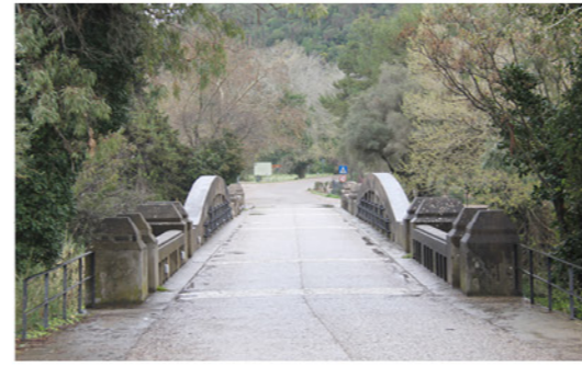
5 The bridge over the Kladeos river
