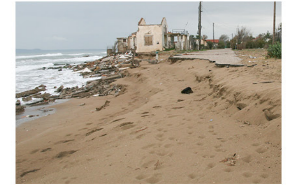
An abandoned illegal second house
