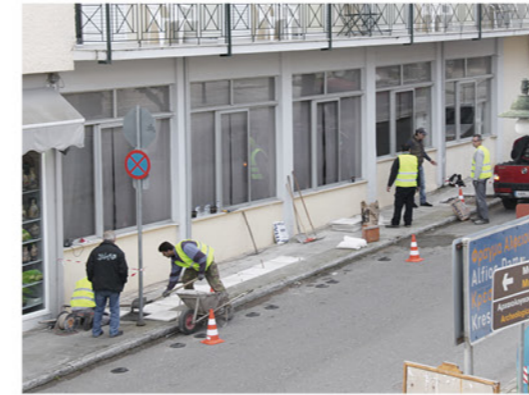
Construction works on the main road preparing for tourist season
