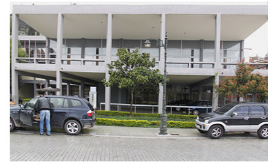
10 The modernist municipality building by Aris Konstantinidis
