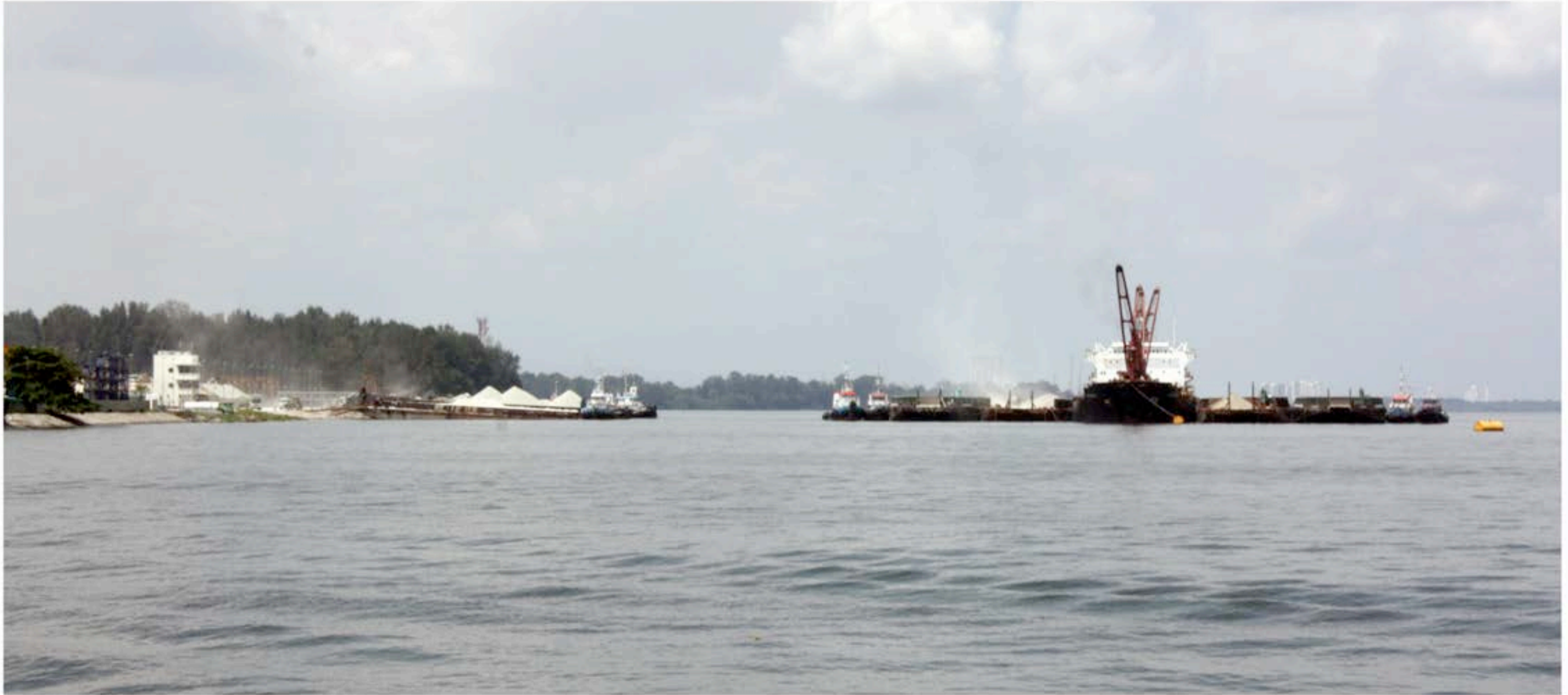
Imported sand arriving at the Pulau Ponggol Timor sand depot by barge
