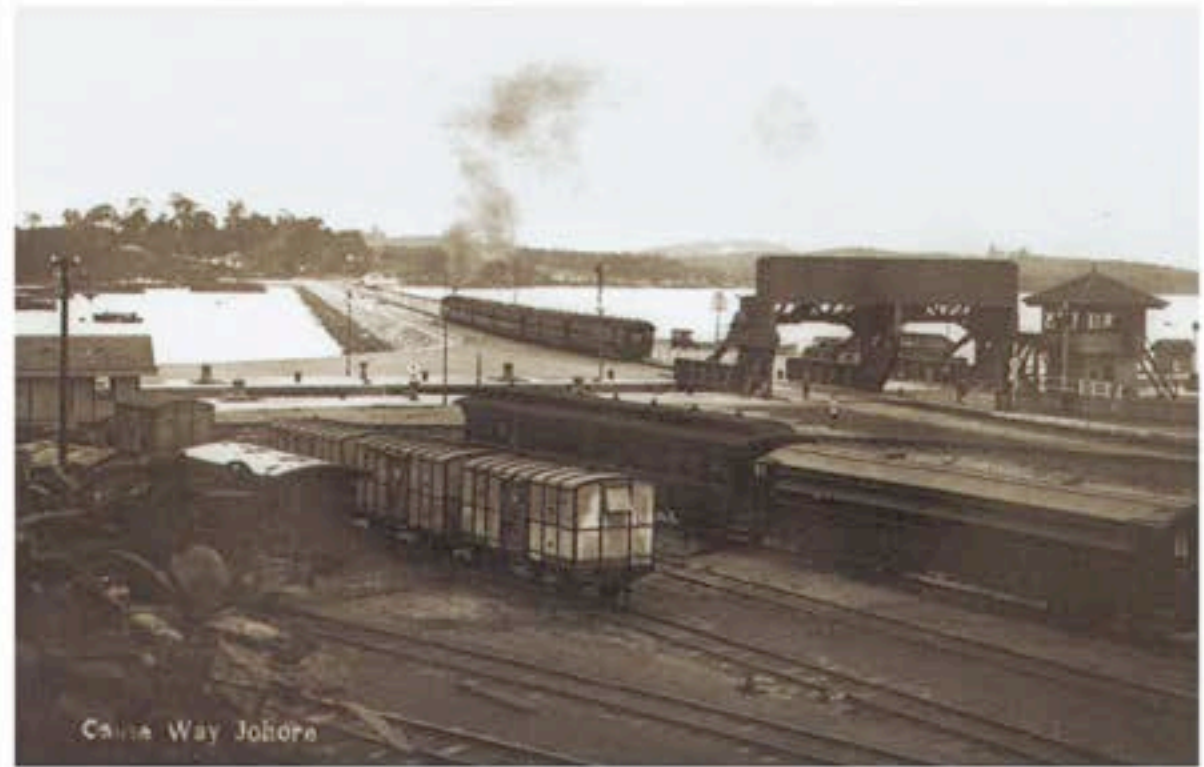
Causeway railroad in Johor Bahru
