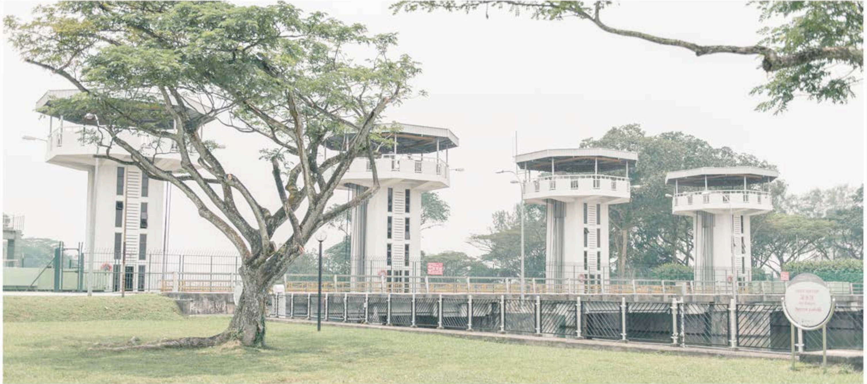
Tide control facility at the dam of the Kranj reservoir
