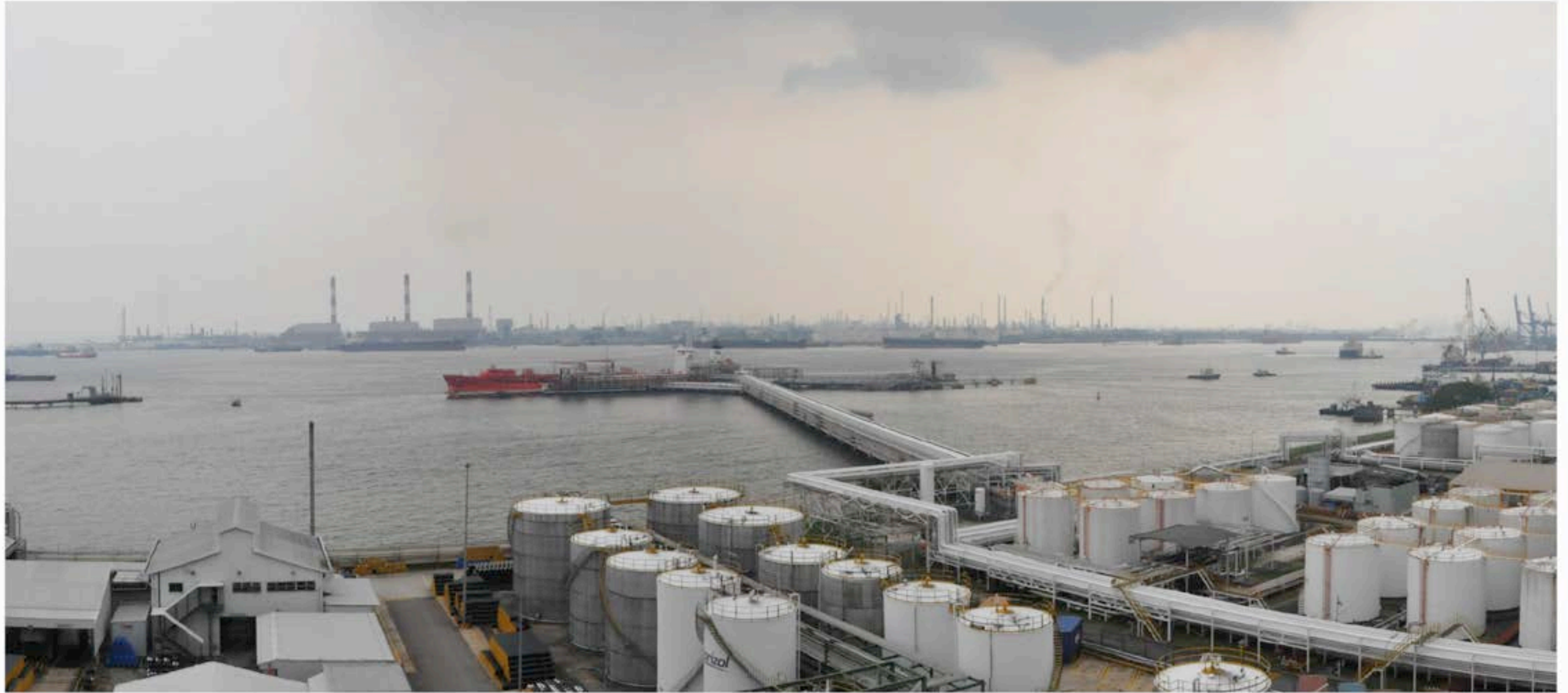
View to Jurong Island from the Vopak jetty in Singapore mainland
