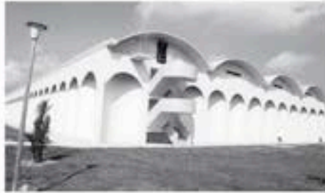
Service Reservoir - Asmara
