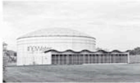
NEWater Plant - Changi
