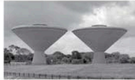
Water Towers - Tampines
