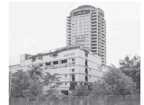
Abandoned Pacific Mall building close to Johor Bahru city center
